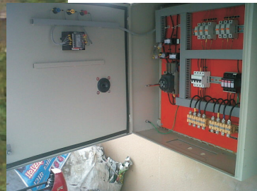
NMC Lakadgaj, Nagpur 25 Kwp
