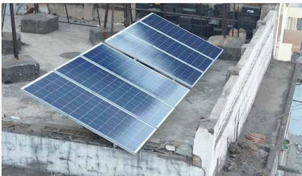
Verma Batteries, Yawatmal 1.7 Kwp
