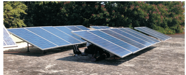
V.N.I.T., (Electrical Engg Dept )Nagpur 5 Kwp
