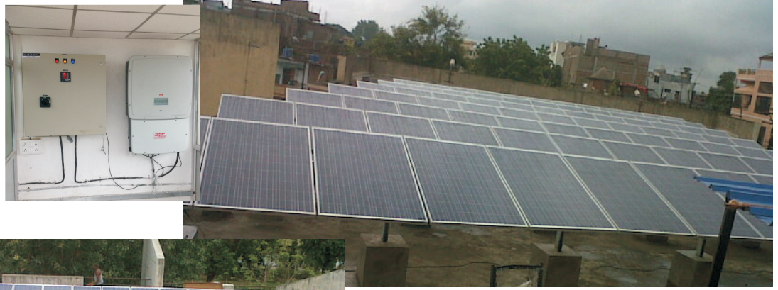
NMC Aashi Nagar, Nagpur 25 Kwp
